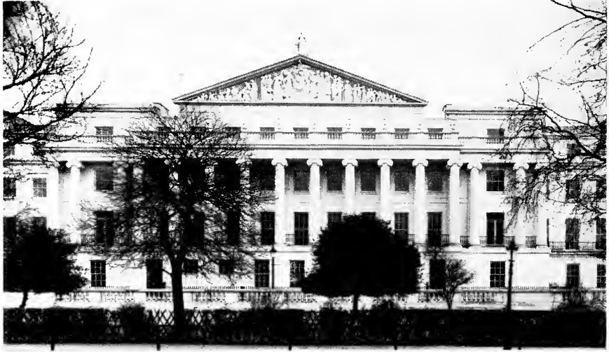
49 and 50. Conservatism. The persistence of the Palladian style in the Georgian Age is equally remarkable. Wanstead House, Essex, by Colen Campbell, begun in 1715, and Cumberland Terrace, London, by John Nash, begun in 1826.
